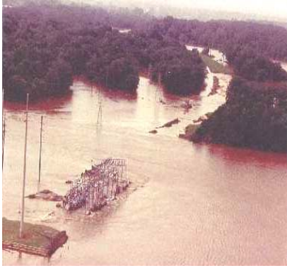
(Source of Photo: Flint River-Georgia Power Company levee failure, Albany, Georgia, September 14, 1994, Georgia Tech)
