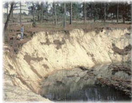
(Source of Photo: Sinkhole in Georgia. Source: USGS.)
